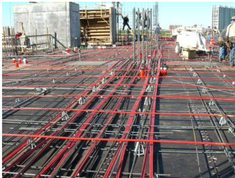
Figure 8: Two-way Post-tensioned tendons prior to casting of concrete. ( www.suncoast-pt.com )
